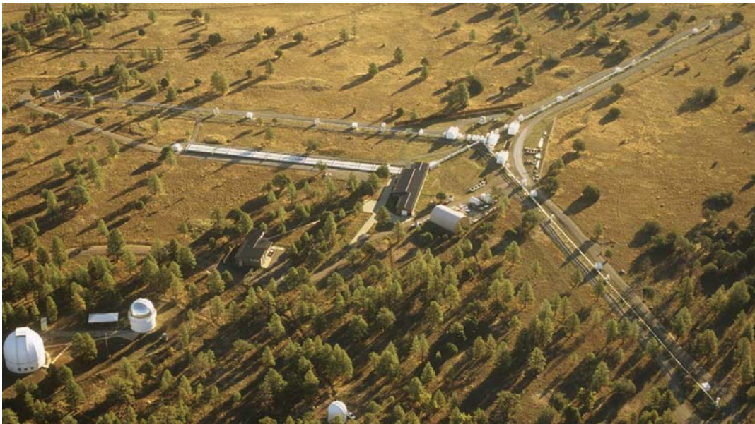
Figure 1. Aerial View of the Navy Prototype Optical Interferometer. (Photo Courtesy of Michael Collier.)
